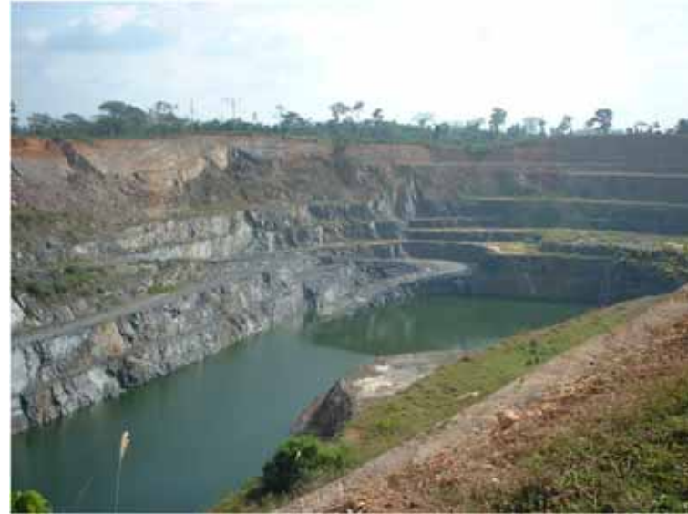
Nkran Pit, Obotan Project
